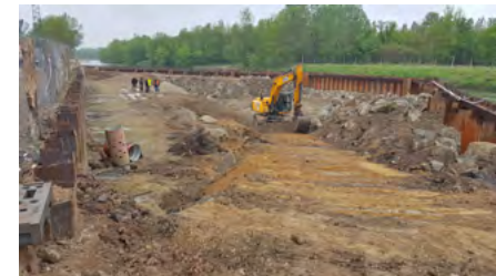
Construction of a Dam on the Dyje River
